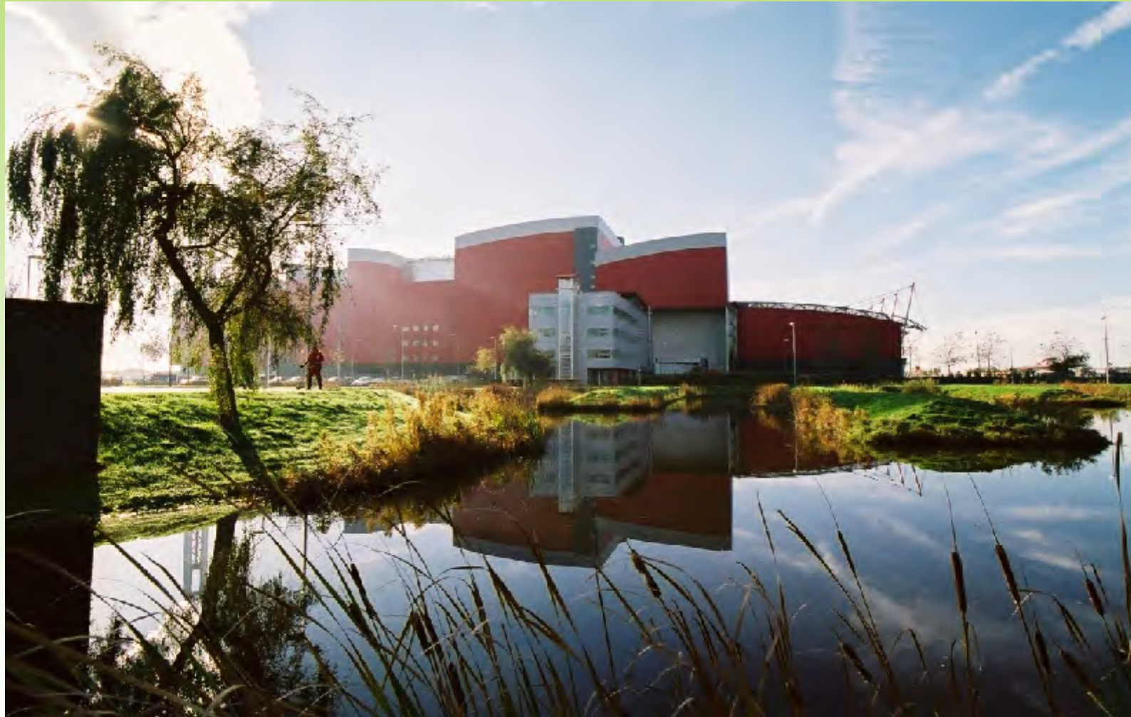
Alkmaar WTE, Netherlands
