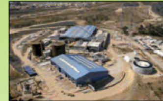
Anaerobic Digestion Plant
