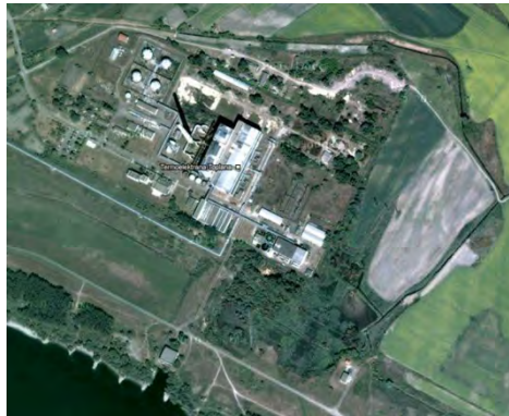
Existing Novi Sad Thermal Power Station
