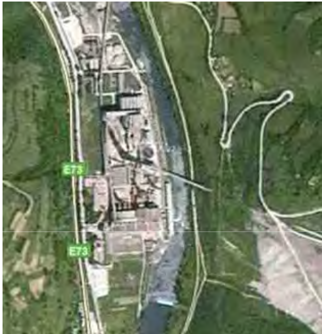
Existing Kakanj Thermal Power Station
