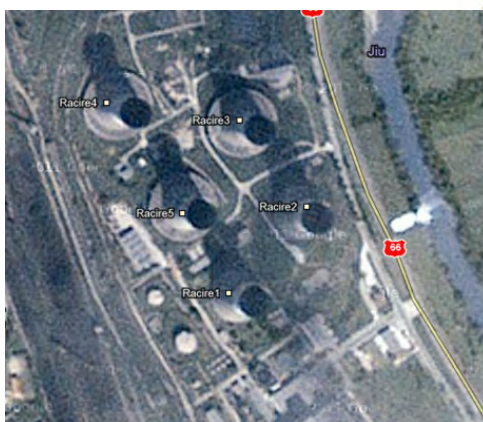
Existing Rovinari Thermal Power Station
